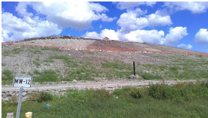
Area with Poor Intermediate Cover
