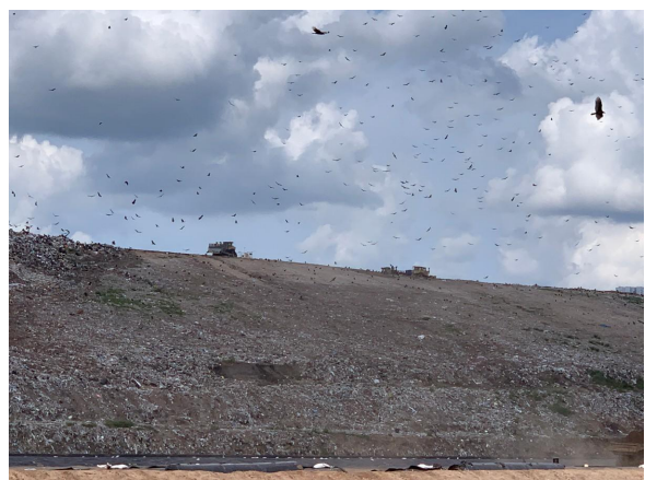
Close-up of inadequate cover
