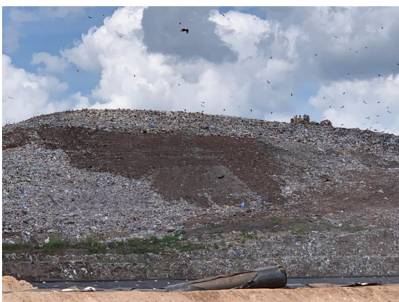
Close-up of inadequate cover
