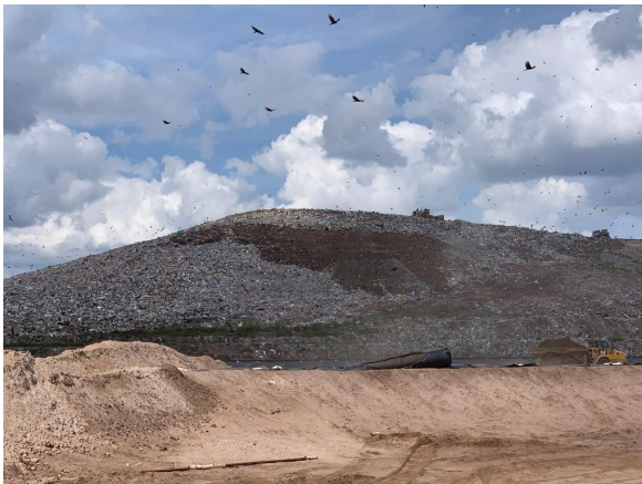
Close-up of inadequate cover
