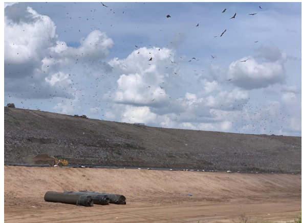
Close-up of inadequate cover
