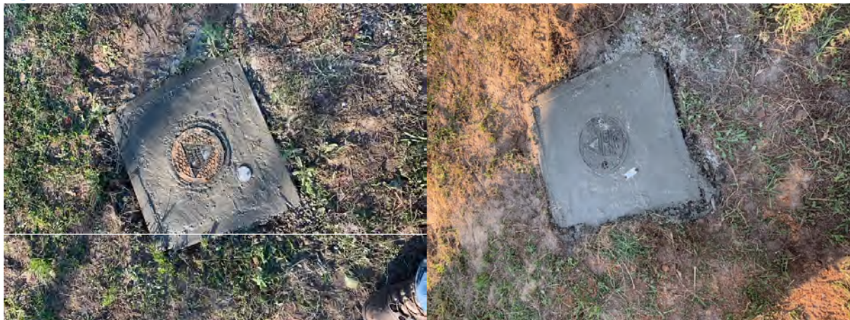
Figure 5: Photos of new well pads on MW-19 and MW-19D
