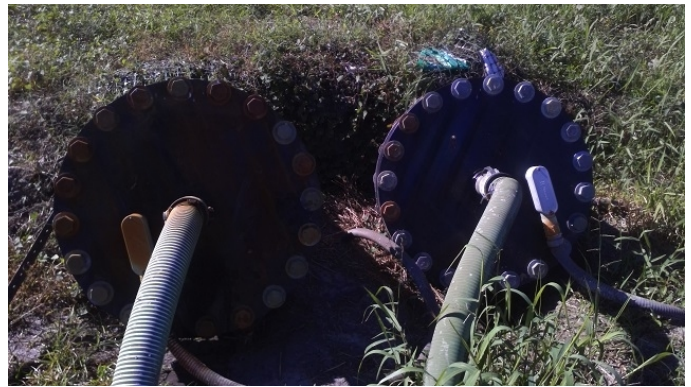
Flex Hose @ Tanks - Poor Cond.
