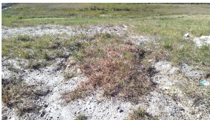
Erosion on Side Slope
