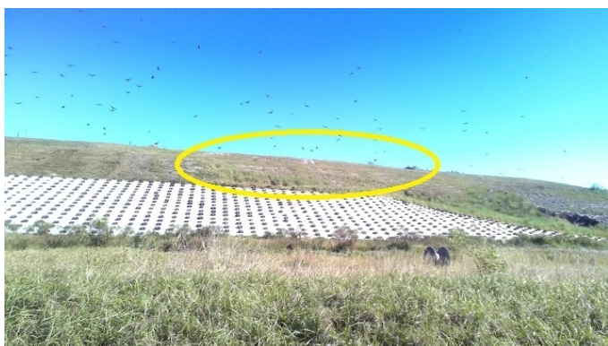
Erosion on Side Slope
