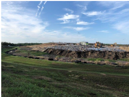
Working face berm
