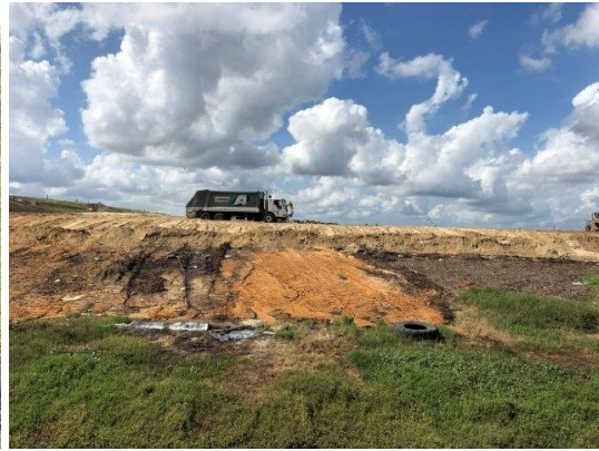
Seep Repaired on Phase III
