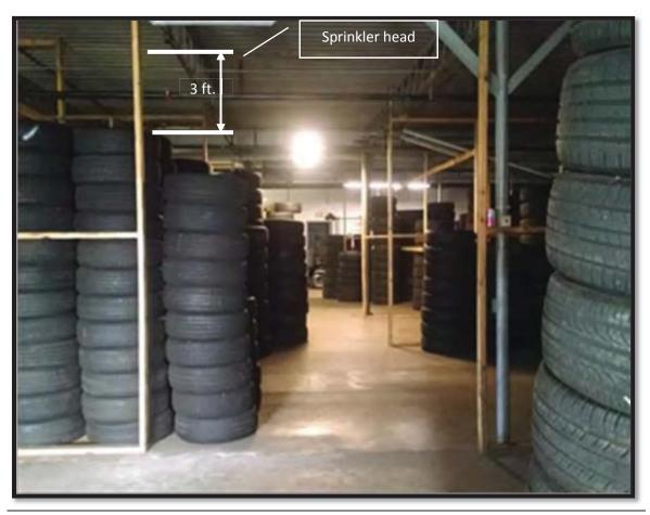
Photo 1 - Sprinkler System Clearance
