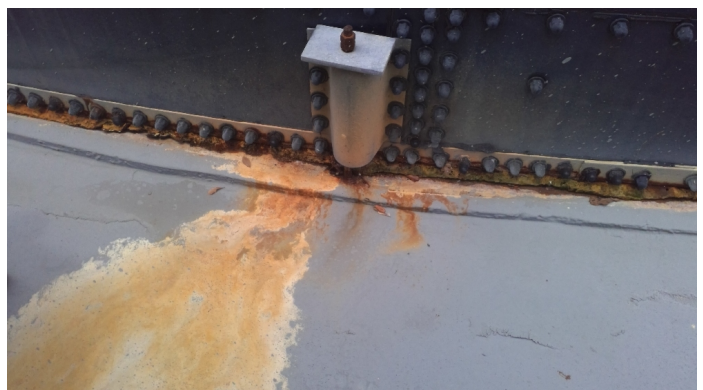
Concrete Floor Staining - T1
