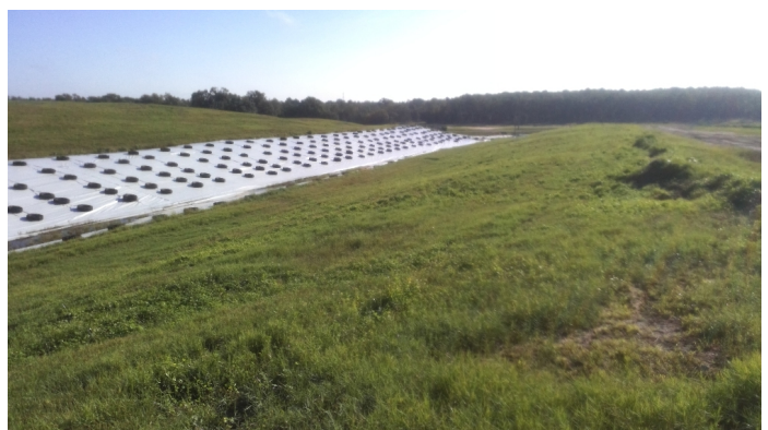
Valley Between SW1 &amp; SW2
