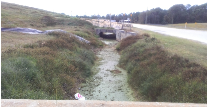
Anchor Trench Tie-In Berm
