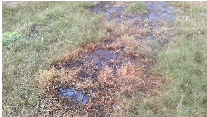
Leachate w/in Perimeter Swale
