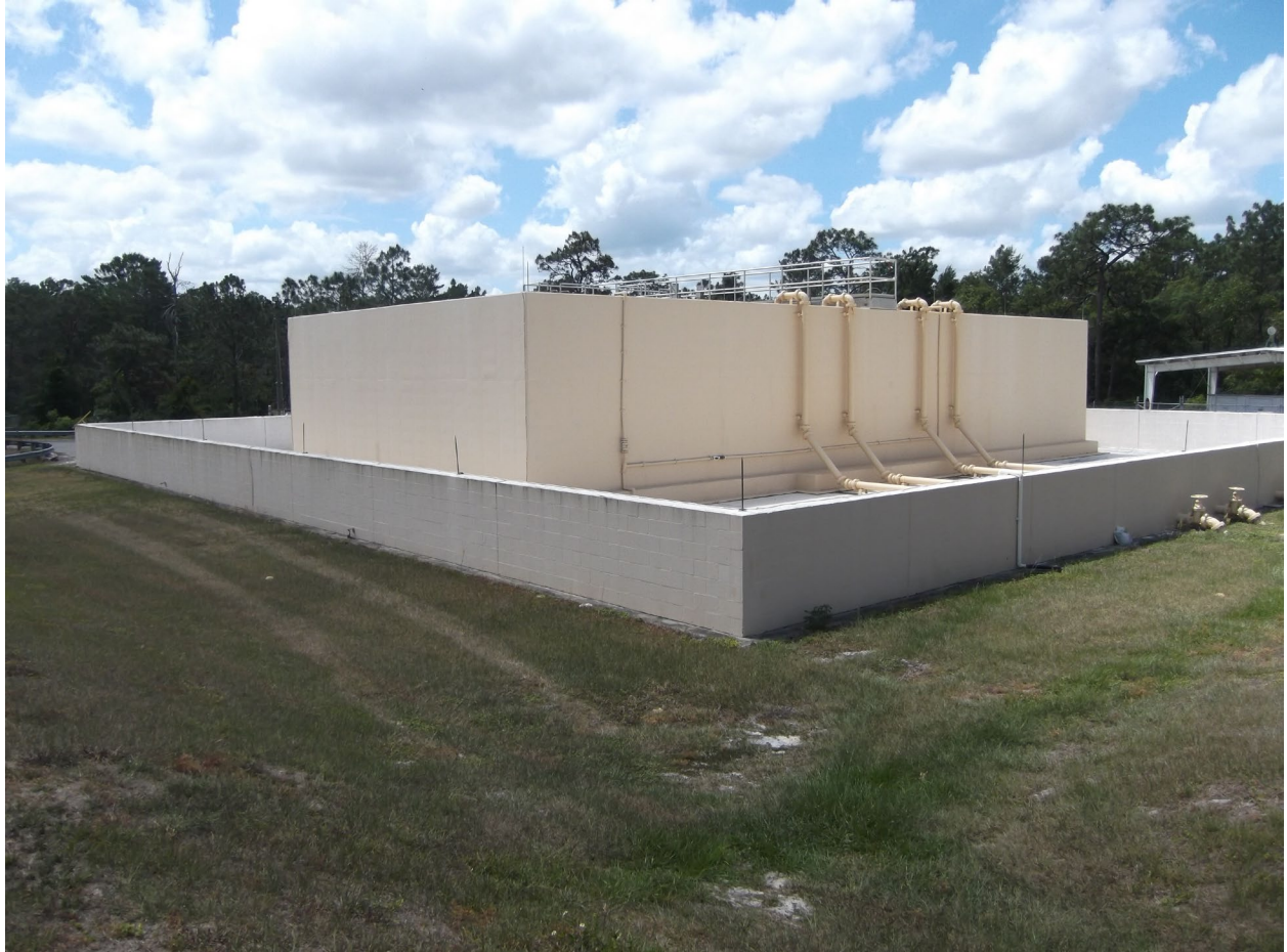
Photo 5: Exterior of the tanks.
