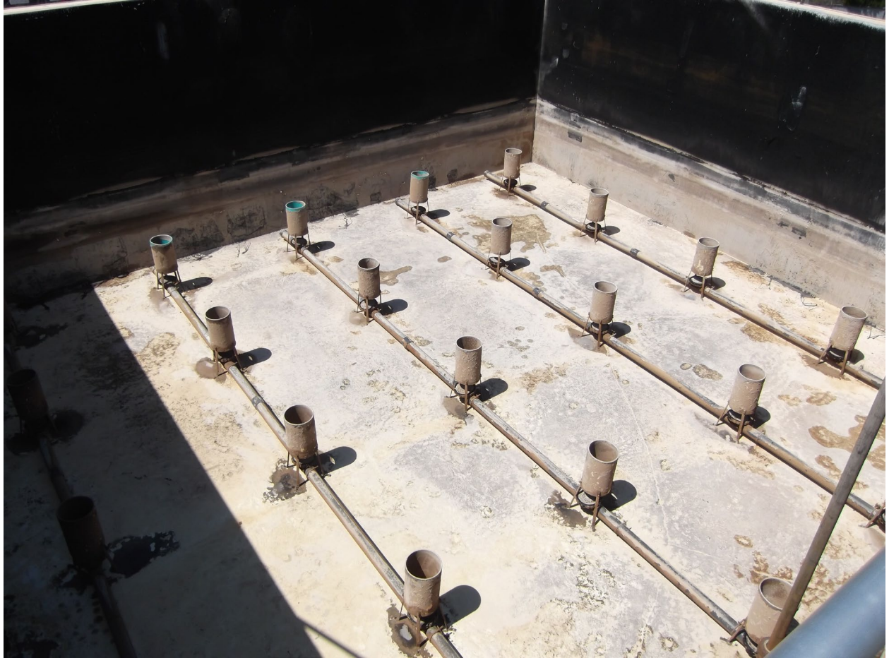
Photo 3: South Leachate Tank after the cleaning and removal of grit.
