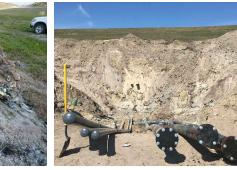
MARCH 2017: TRENCHING TO TOP OF CLAY FOR PHASE I HEADER -APPROXIMATELY 35 FEET (HORIZONTALLY) FROM THE TOP OF THE CONTAINMENT BERM MARCH 2017: CONNECTION TO THE PHASE I HEADER AND LATERAL PIPES AT THE TOP OF CLAY - APPROXIMATELY 50 FEET (HORIZONTALLY) FROM THE TOP OF THE CONTAINMENT BERM
