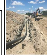
APRIL-MAY 2018: TRENCHING TO TOP OF CLAY FOR THE 2-4 IEADER - APPROXIMATELY 50 FEET (HORIZONTALLY) FROM THE TOP OF THE CONTAINMENT BERM
