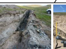
APRIL-MAY 2018: TRENCHING TO TOP OF CLAY FOR THE 3-1 HEADER - APPROXIMATELY 50 FEET (HORIZONTALLY) FROM THE TOP OF THE CONTAINMENT BERM
