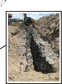
JUNE-JULY 2017: TRENCHING TO TOP OF CLAY - PHASE II CUTOFF TRENCH - APPROXIMATELY 35 FEET (HORIZONTALLY) FROM THE TOP OF THE CONTAINMENT BERM
