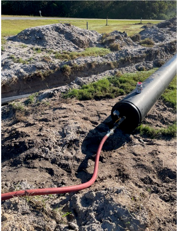
Pressure Testing Header Lines
