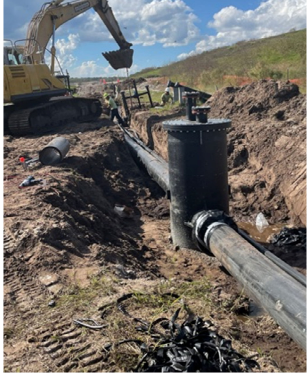
16-inch Header Connection with CS-12
