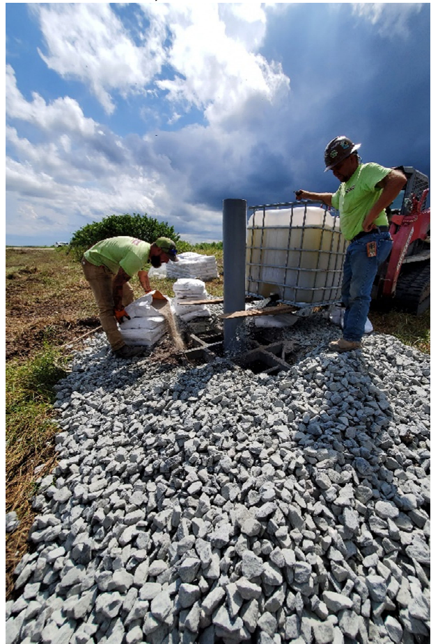
Vertical Well Installation
