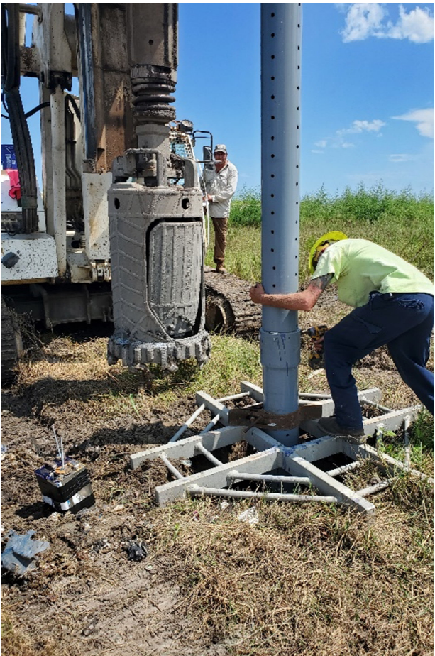
Vertical Well Installation
