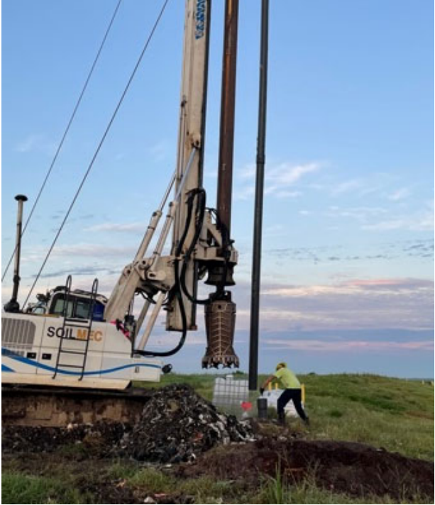
Vertical Well Installation
