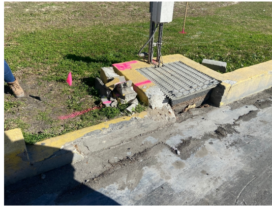
WTE - Ash Building Curb Damage
