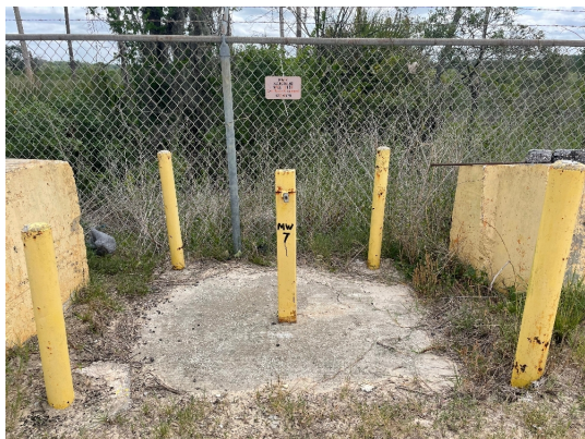
MW-7 Cracked Pad
