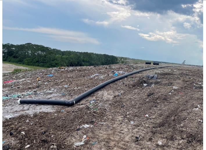
Solid and Perforated Pipe Prepped for Placement
