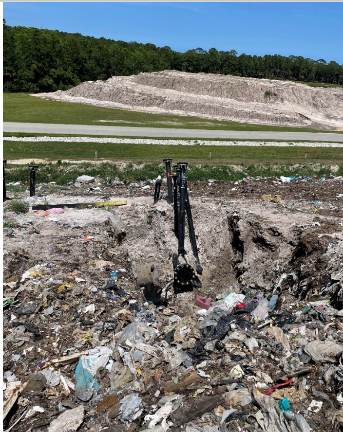
HC-23A, tie-in to header area exposed
