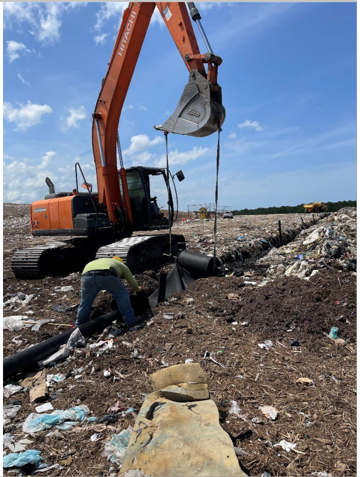
Geotextile fabric over HC-23A
