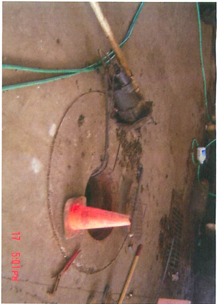
- Leachate Pump pulled out
