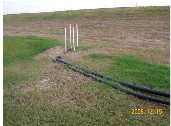
LCS piping from TPS-6 into system
