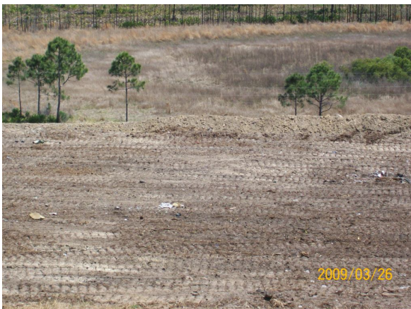
Inadequate initial cover.
