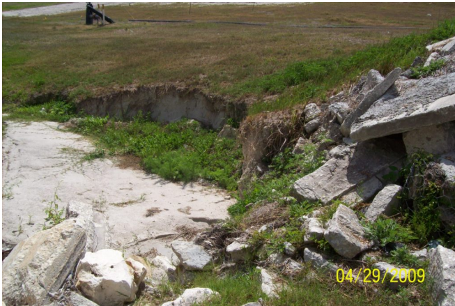
stormwater ditch (nw corner)
