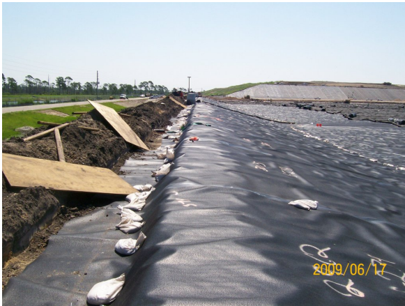
phase II, cell II, LCS trench (N)
