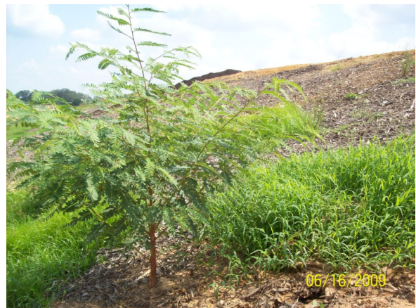
Tree on side slope.
