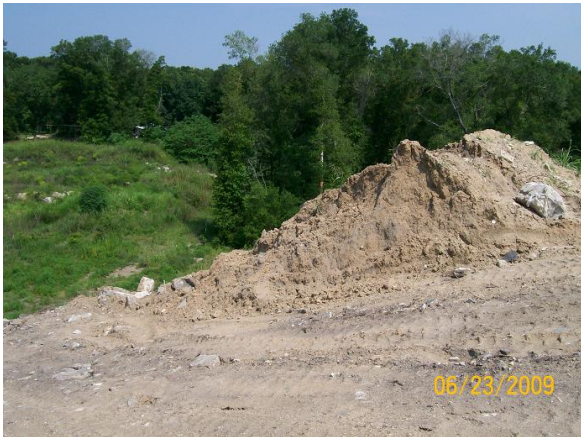
Slopes being corrected to 3 to 1
