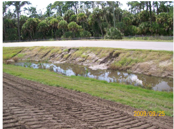
Erosion @ W stormwater swale
