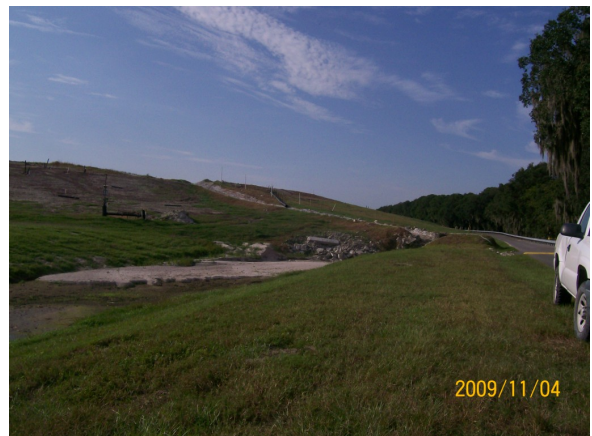
sedimentation in SW ditch
