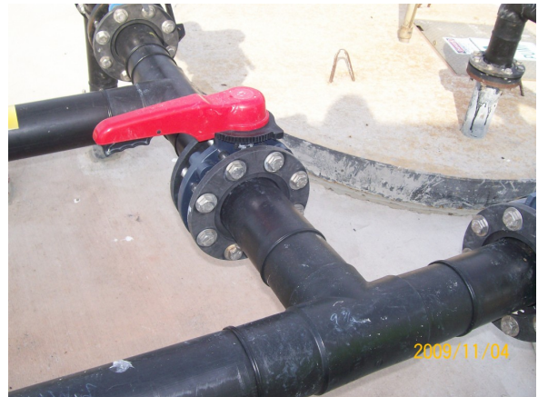
PPS-B to PPS-A bypass valve
