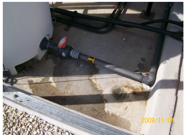
effluent tank, sulfuric "drip"
