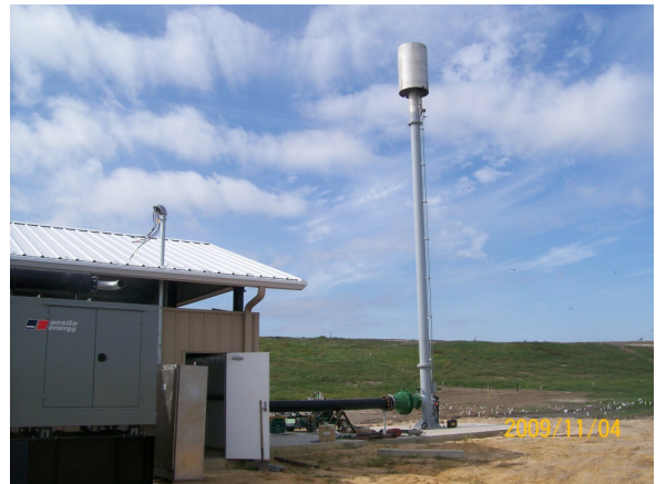
gas flare construction
