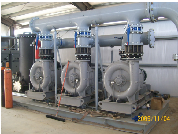
LF gas blower construction
