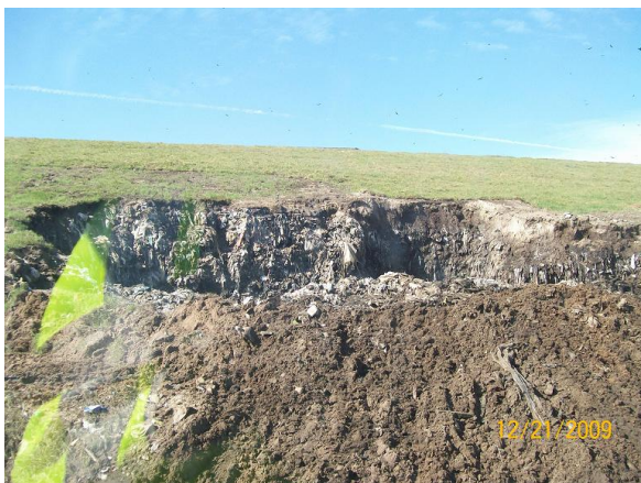
Leachate Seeps Being Repaired
