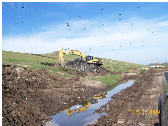
Leachate Seeps Being Repaired
