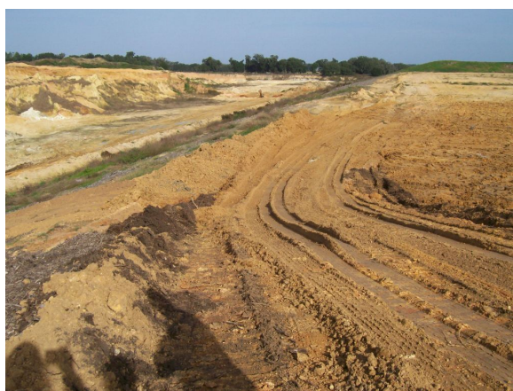
W slope, looking N
