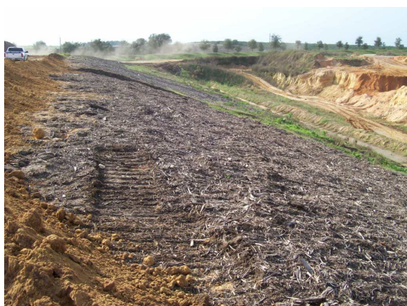
W slope, looking S
