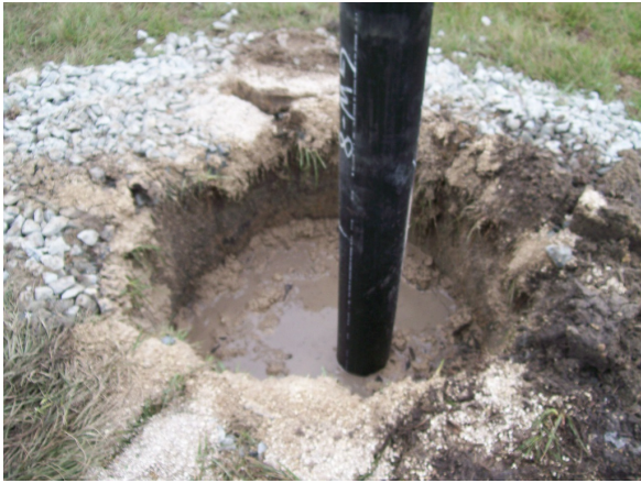
GW-8 installation, bentonite plug
