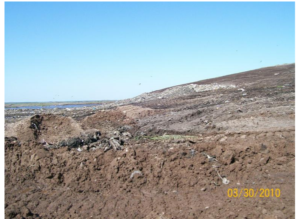
2nd Working Face Area
