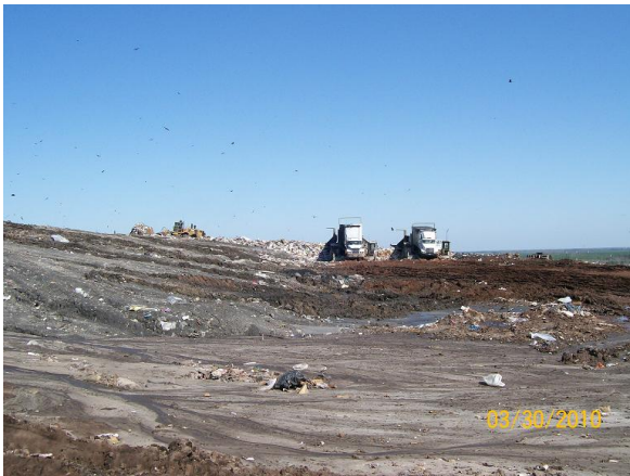
Bottom of Working Face
