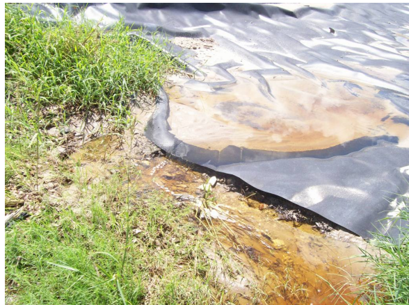
Phase V - lined ditch to flume
