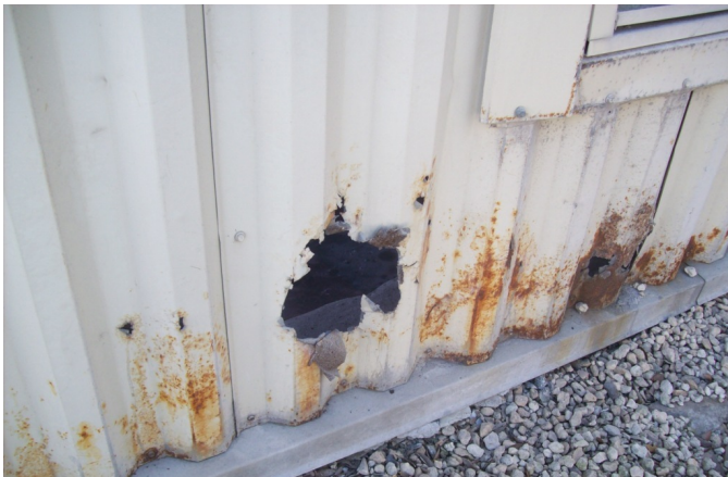
Damage on ash building facade
