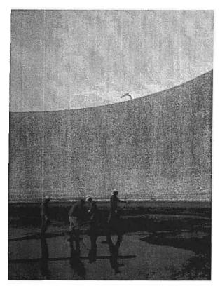
Figure 5 – CECS crew cleaning the tank floor.
