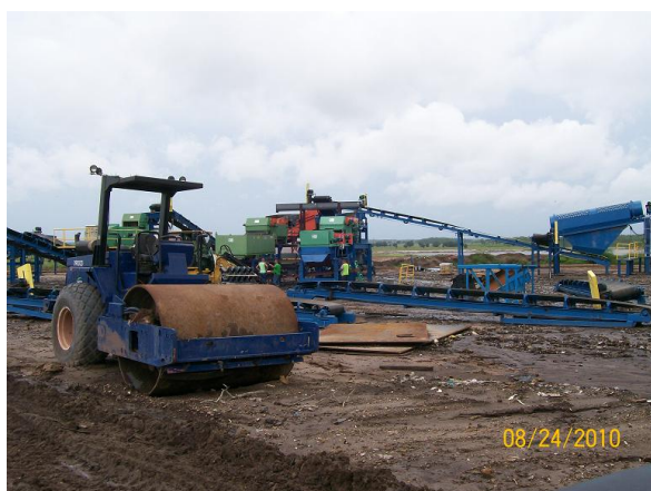
Construction of Auto Fluff Area
