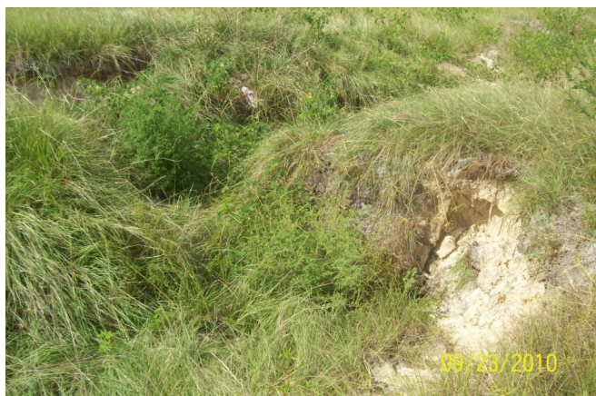
Erosion, N slope, E conveyance
