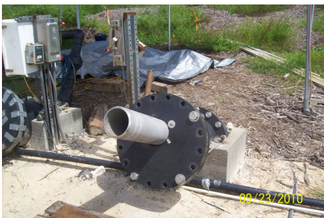
Slip-lined LDS riser pipe
