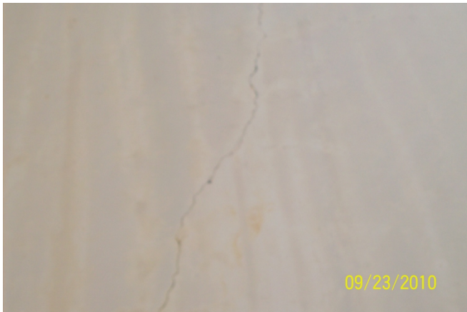
Surface cracks, leachate tank
