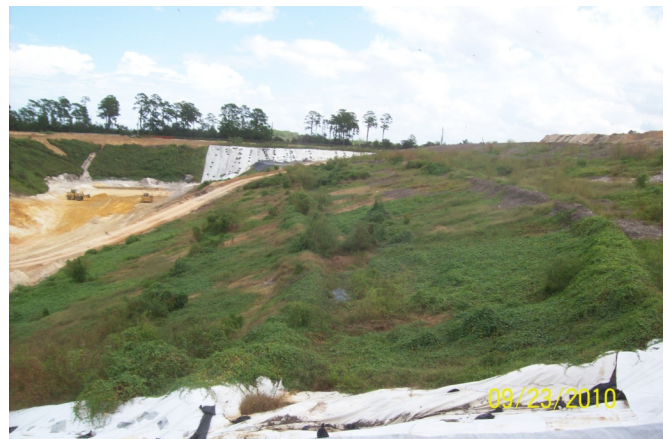
Ponding, N slope Phase II
