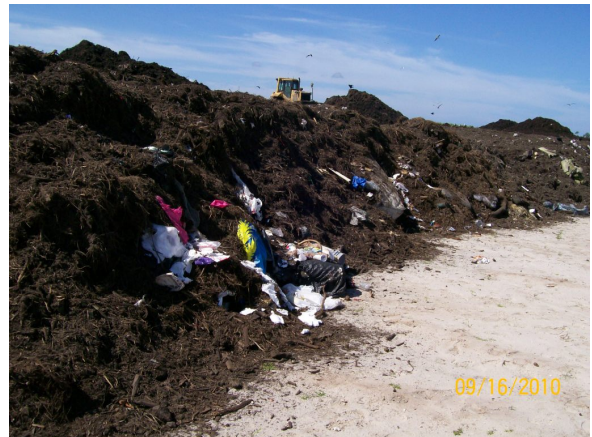
Phase II, select layer cover thin
