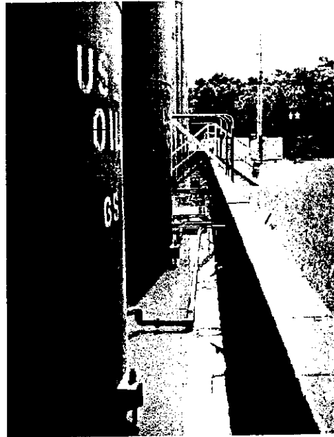
Figure 3. Water in secondary containment
