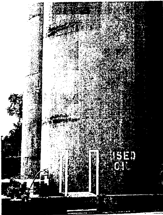
Figure 6. Float indicates tank contains waste
