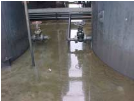
9. Oily wastewater in tankyard secondary containment
