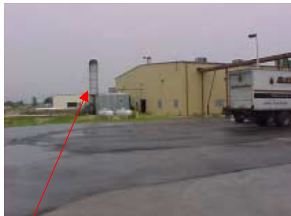
12. Oxidizer tower for burning off excess hot gas
