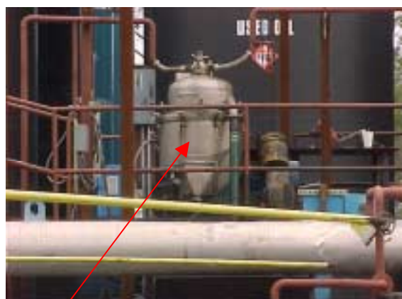
10. Centrifuge for mechanical removal of solids before thermal processing (not yet in use)
