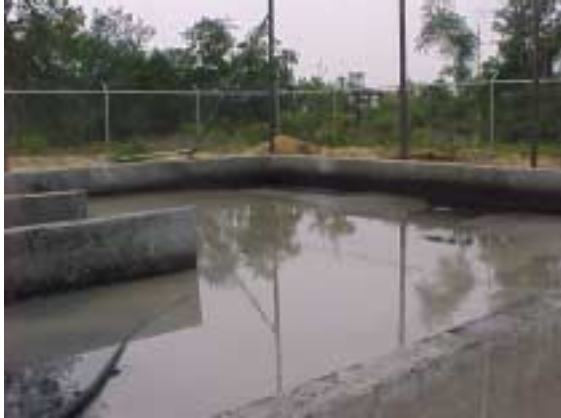
13. Solid waste treatment pit currently under construction
