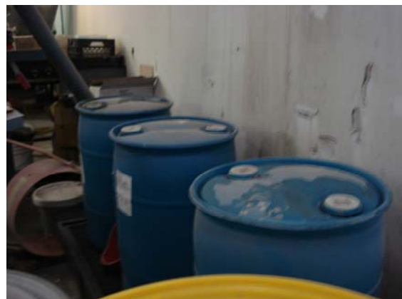
Figure 10: Satellite area for batteries
