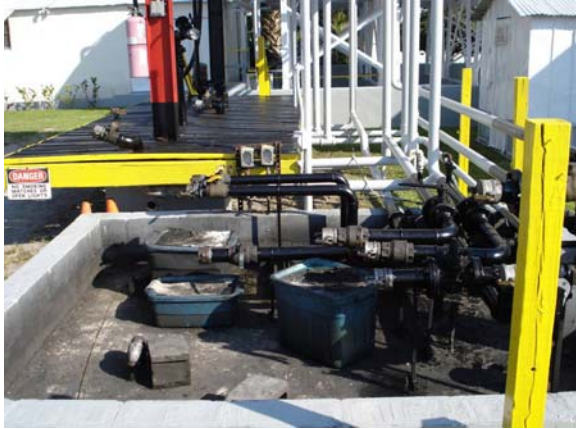
Figure 1. Loading Manifold
