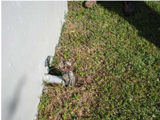
Figure 5. Containment discharge pipe locked
