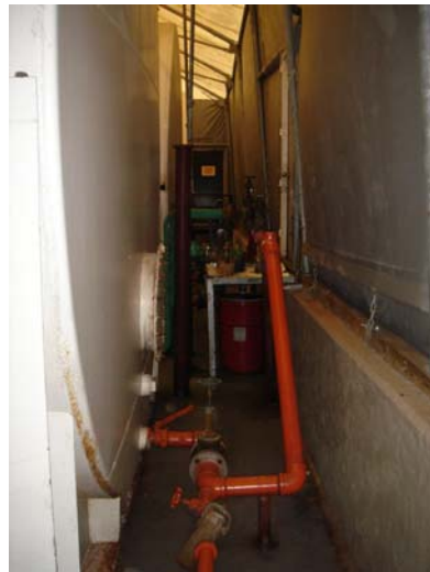
West end of tank Farm
