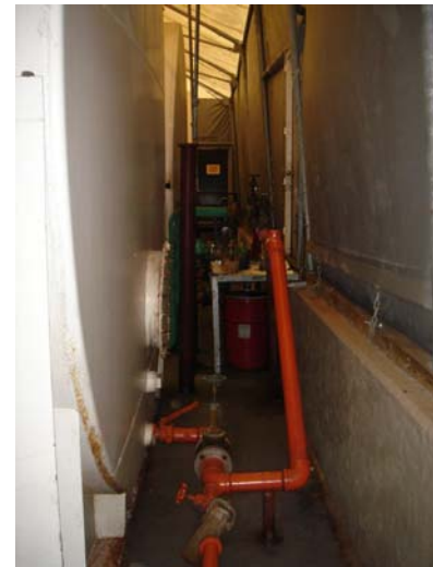
West end of tank Farm
