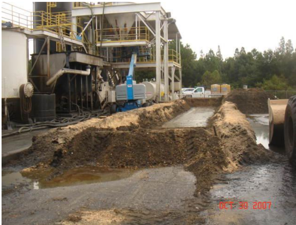
Cone Bottom Tank, Stabilization pad
