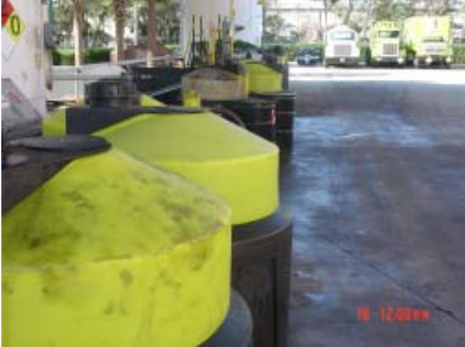
Figure 9: Temporary antifreeze storage
