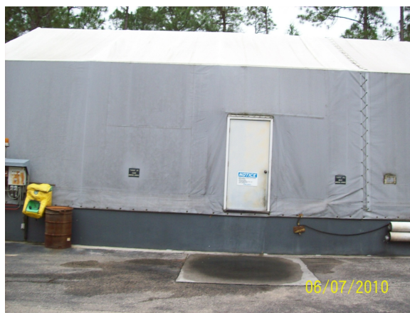
D. Tank Storage
