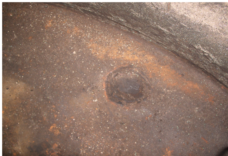
9P Tank - Internal Floor Patch Plate Photo
