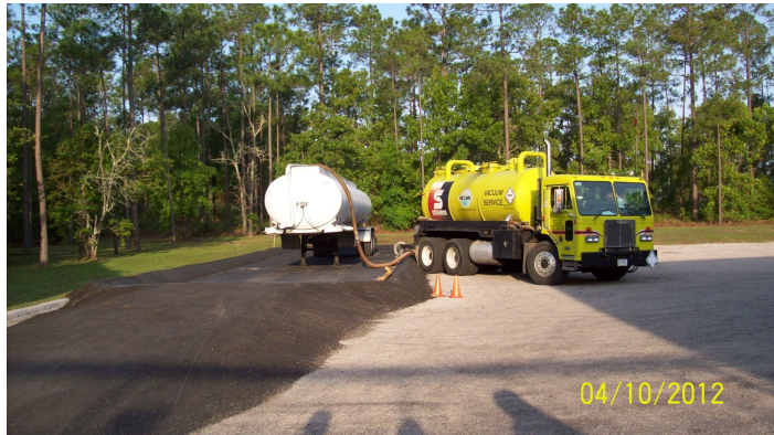
Secondary Containment for tanker
