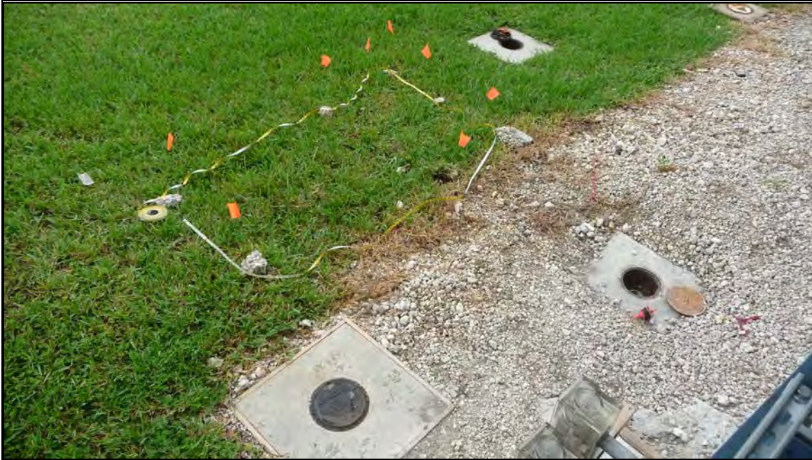
Figure 1: View of excavation area
