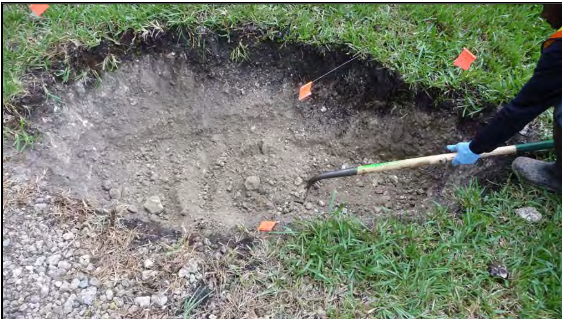
Figure 8: Digging at estimated 2 ft bls
