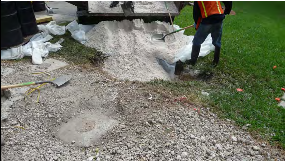
Figure 11: Backfilling with masonry sand (previously tested for arsenic)
