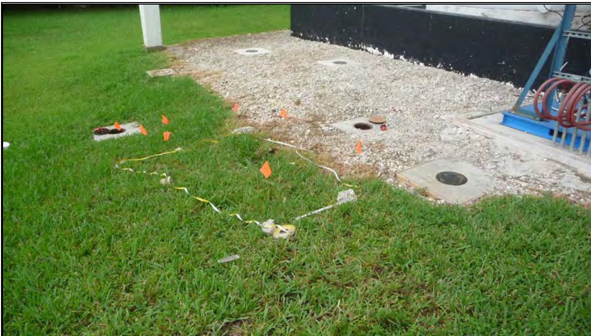
Figure 2: Alternate view of excavation area
