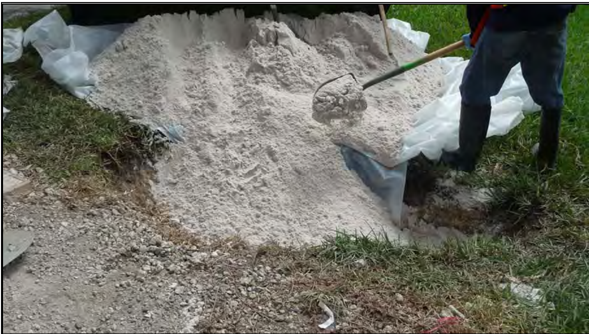
Figure 12: Continue backfilling the excavated area
