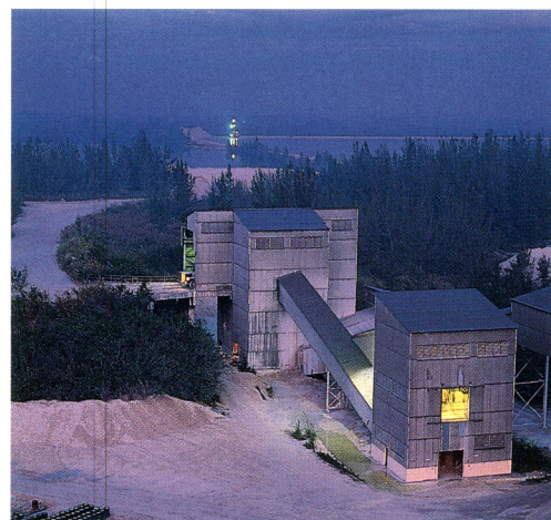
The rock is crushed and conveyed to our cavernous materials storage building.
