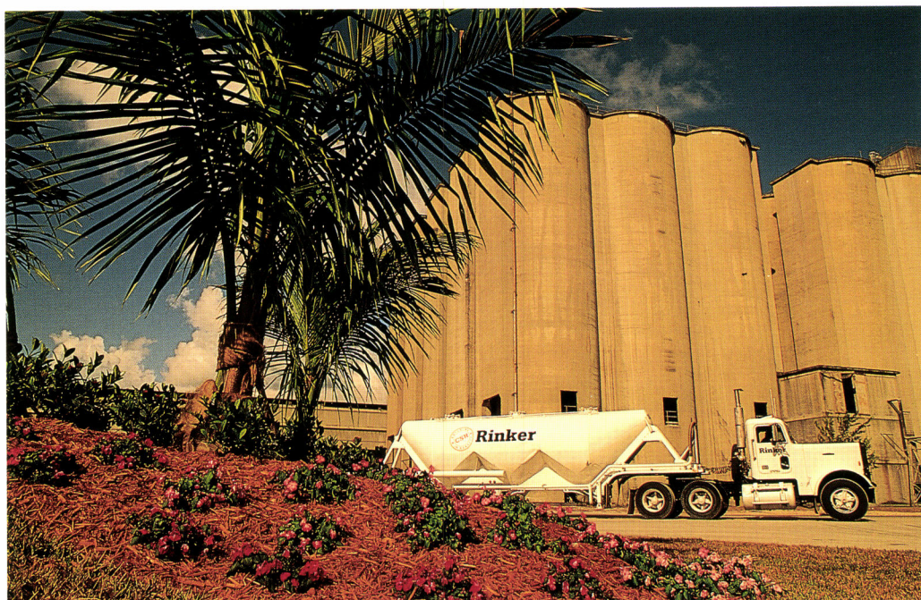
Tank trucks are filled from our 30 storage silos, each with a capacity of 2,500 tons.
