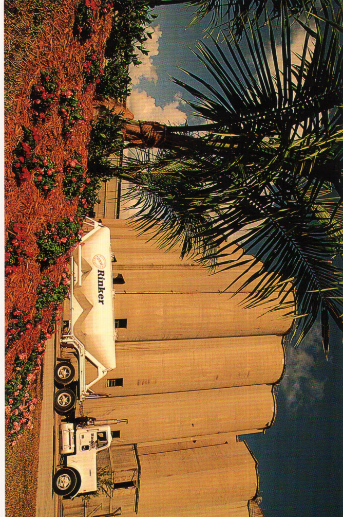
Tank trucks are filled from our 30 storage silos, each with a capacity of 2,500 tons.
