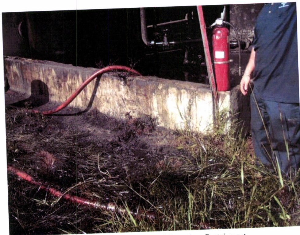
5 of 18: Spill at NE Corner of Secondary Containment
