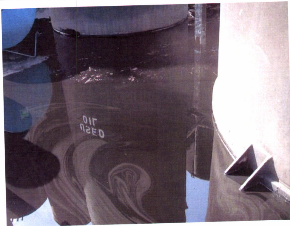
1 of 18: Oil in secondary containment.
